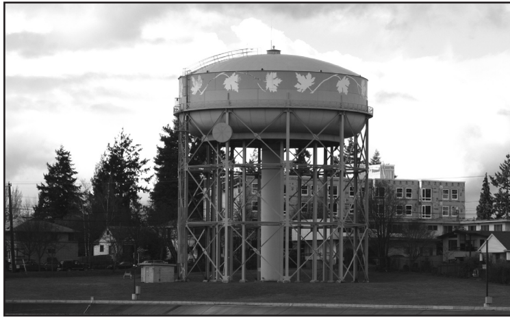
• The Maple Leaf water tower & reservoir near Roosevelt and NE 85th •
